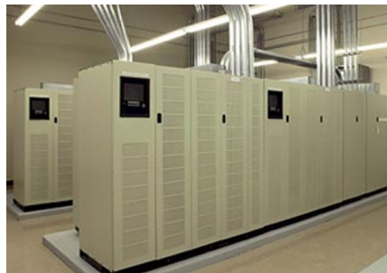
Uninterrupted Power Supplies
