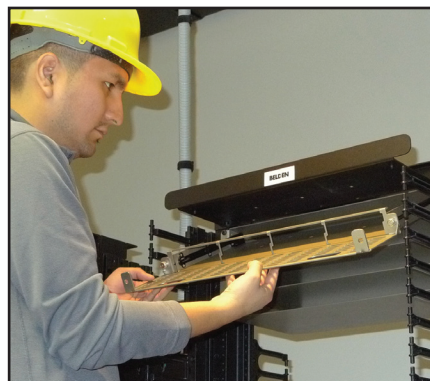
Slide-in trays tilt outward to improve accessibility.
