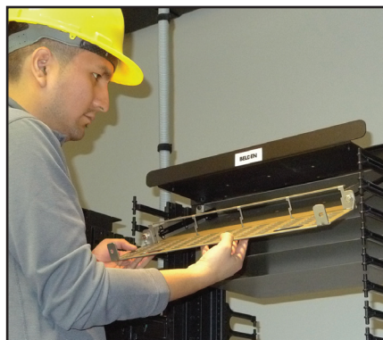
Slide-in trays tilt outward to improve accessibility.
