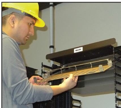
Slide-in trays tilt outward to improve accessibility.
