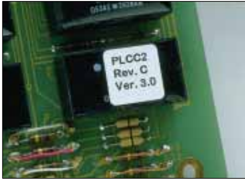
Circuit Board Labeling
