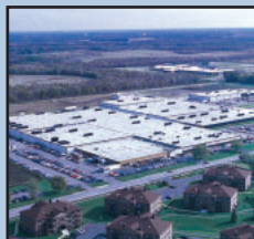
PANDUIT Corp. Worldwide Headquarters Tinley Park, Illinois 60477-3091
