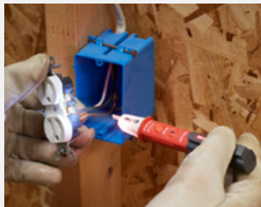
Test wires for AC voltage
