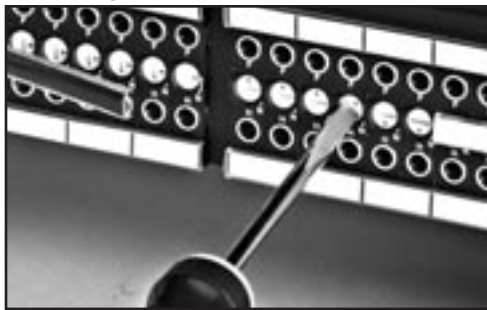
Center Strip Removes For Normaling Access
