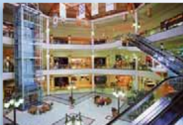
■ Building Management Systems
