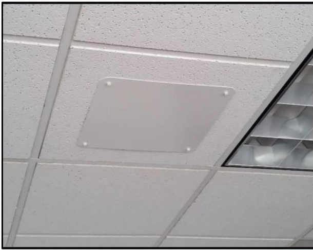
Installed Antenna
