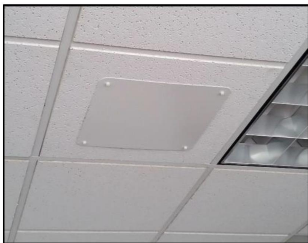
Installed Antenna
