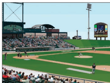
Ball Park – outdoor system connections
