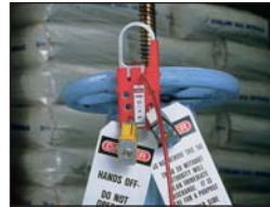
Lockout gate valves
