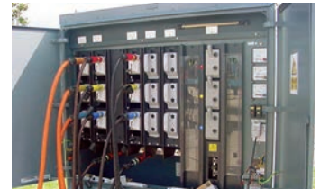
Fuse carriers with integrated PowerLock connectors provide a safe & efficient connection to a power distribution board.
