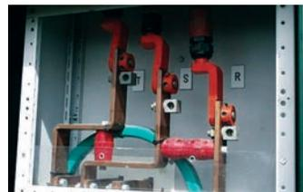
Insulated rotary clamps provided a compact connection to slotted busbar
