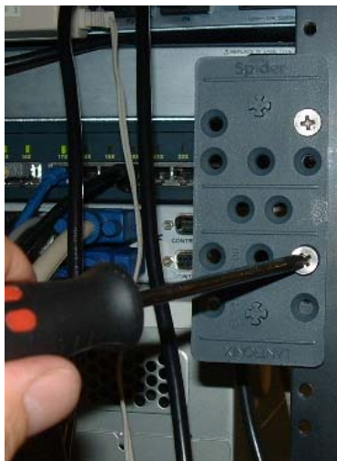
1. Mount the bracket with a Phillips-head screwdriver
