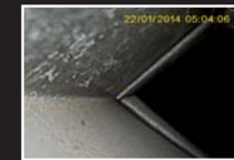
Internal duct work using 28mm detachable camera head (VSC28)
