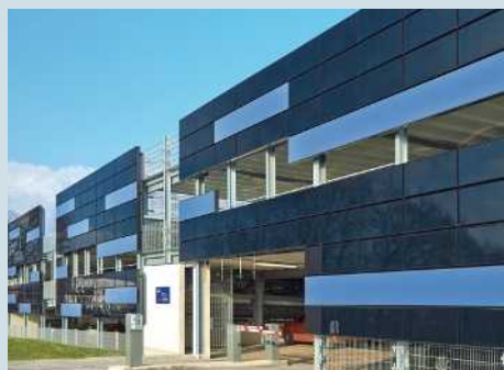
Building-integrated photovoltaics (BIPV)
