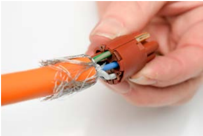
Step 12 - Position shield as shown back over the cable
